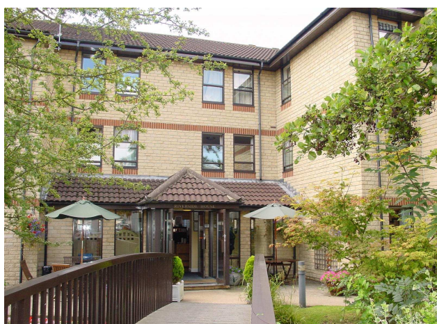
Entrance to Riverside House
